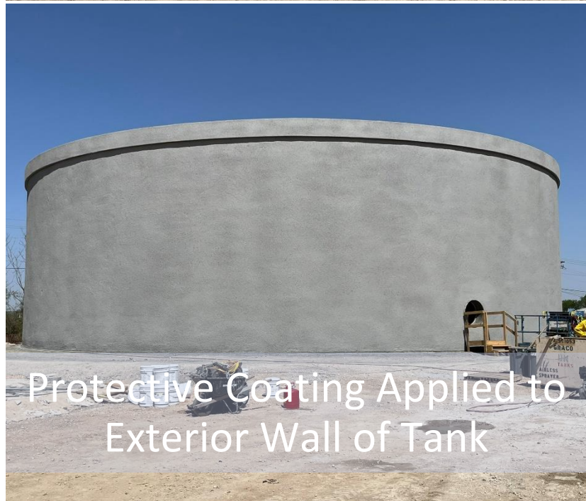
Final Layer of Shotcrete Applied to Exterior Wall of Tank
