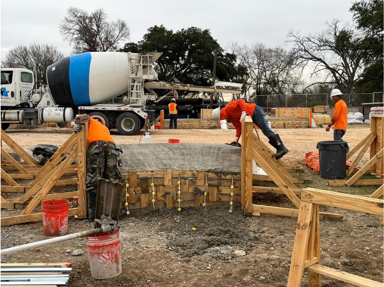
20 – Troweling concrete at Dome Roof Panel piece.
