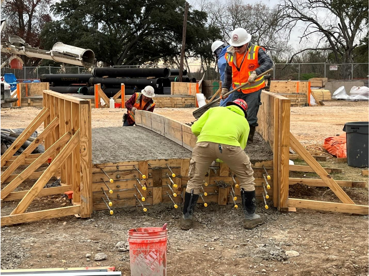
2N – Screeding of concrete at Dome Roof Panel piece.
