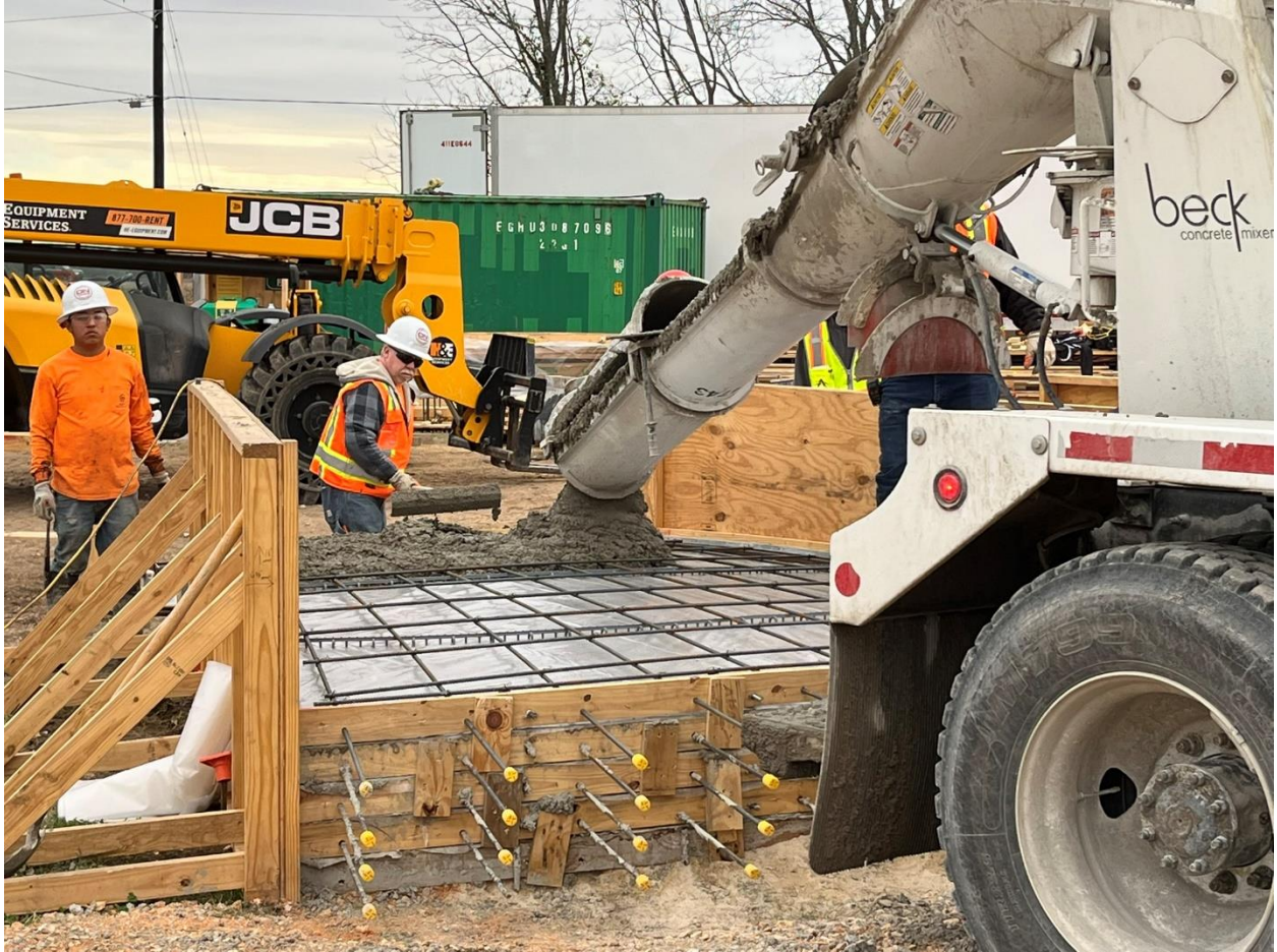
2L – Concrete pour at reinforced Dome Roof Panel piece.
