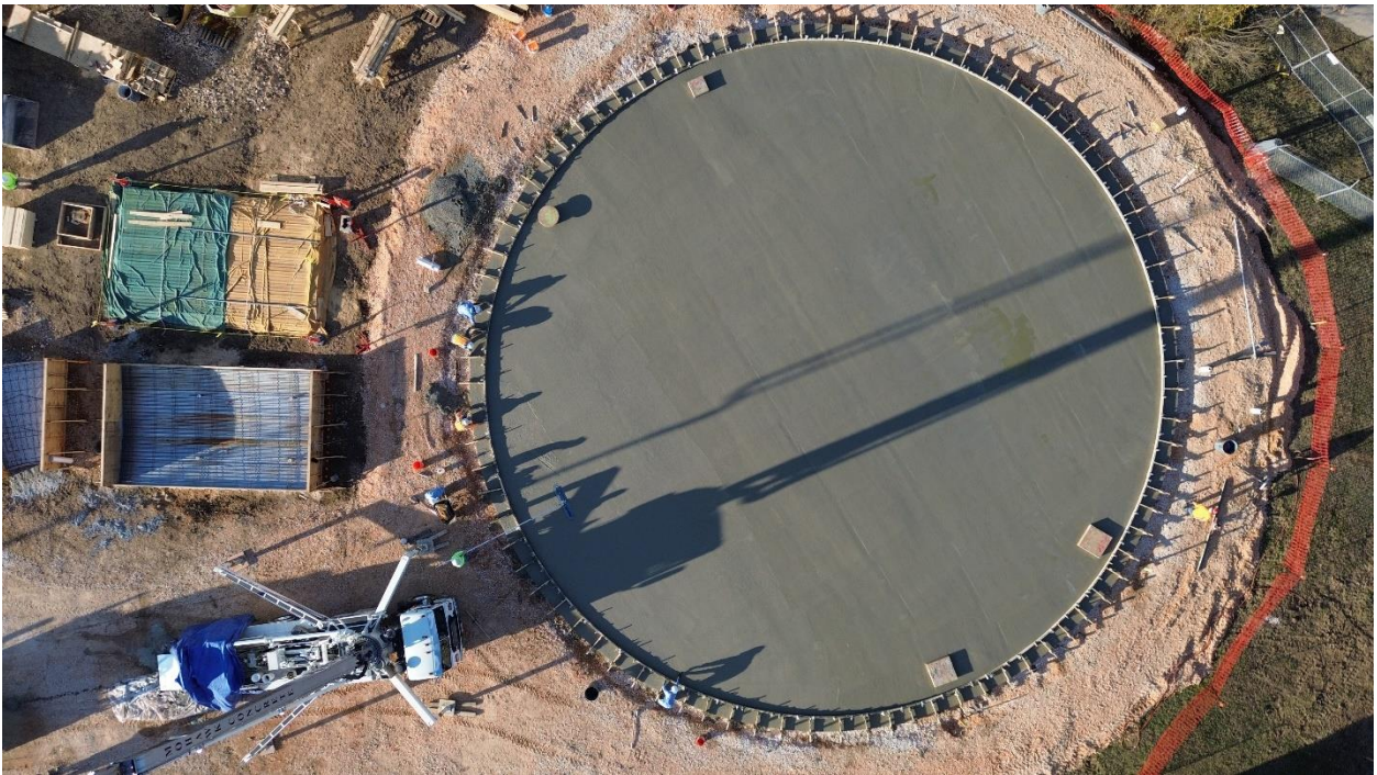
2B – Completed pour of concrete at Tank Floor Structure.
