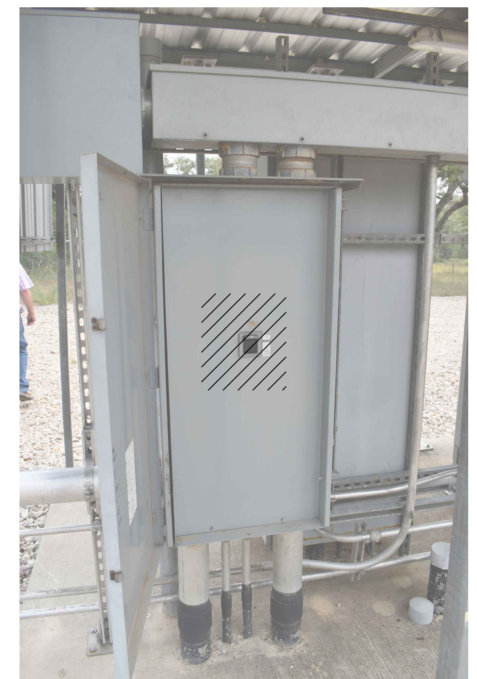
EXISTING 500A MAIN CIRCUIT BREAKER - EXTERIOR
