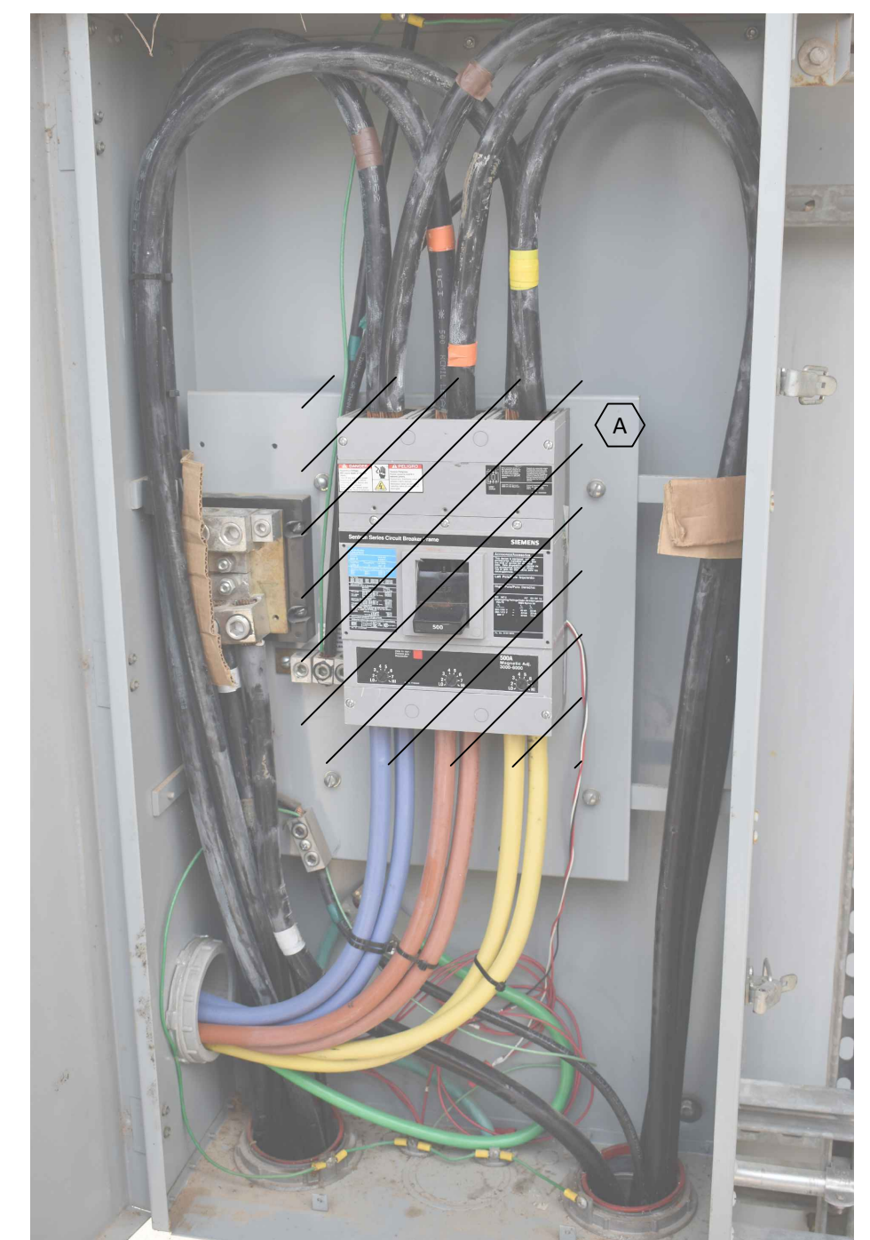
EXISTING 500A MAIN CIRCUIT BREAKER - INTERIOR
