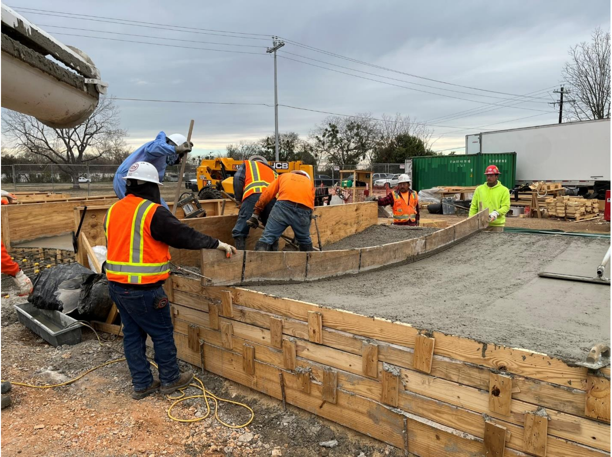
21 – Screeding and floating of concrete for Wall Panel pieces.
