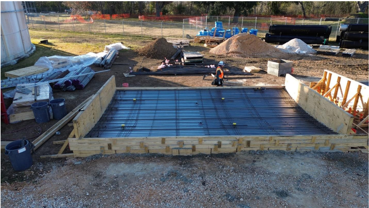
2F – Form with steel panel and reinforcing steel for casting of Wall Panel.
