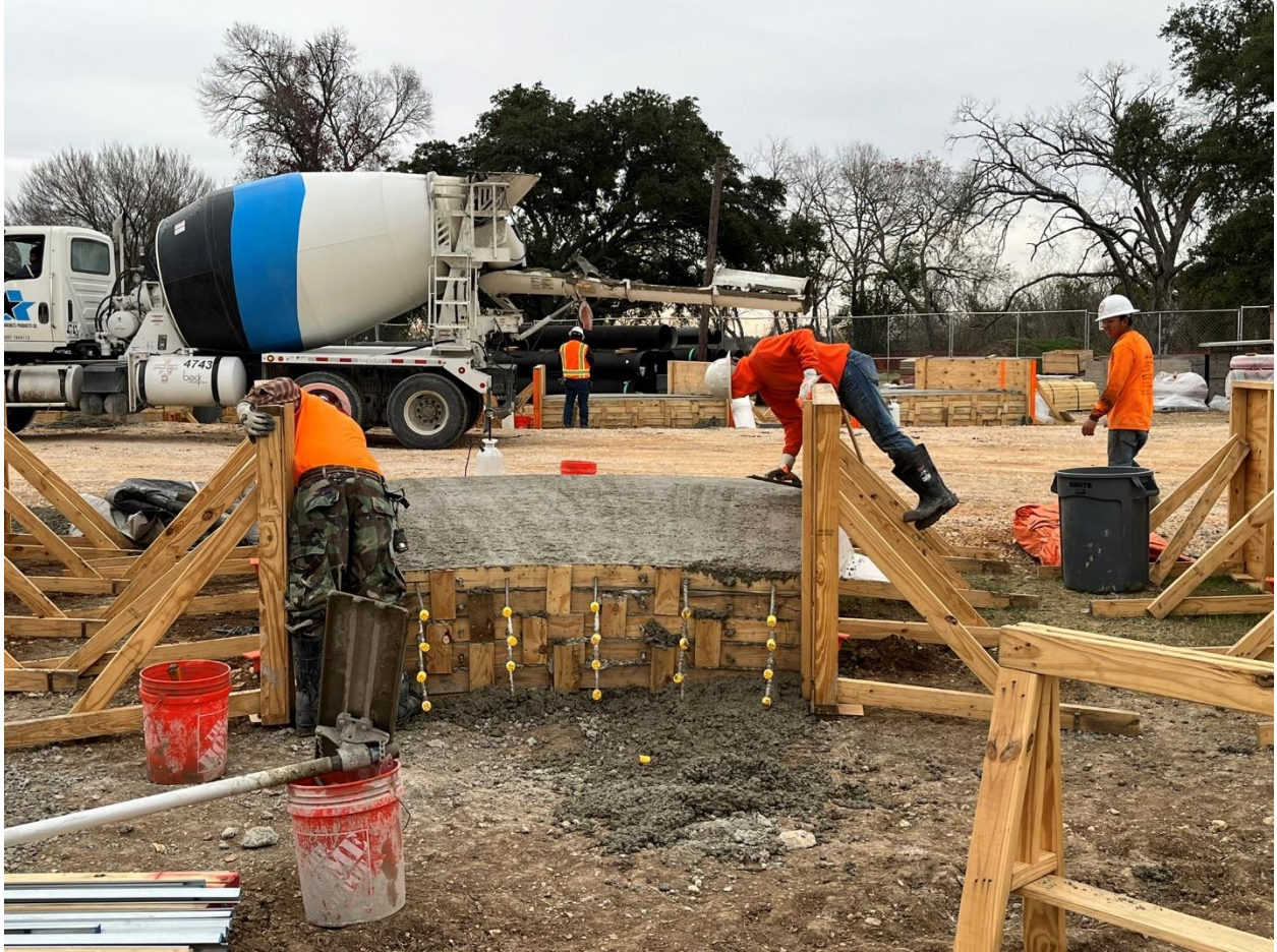
20 – Troweling concrete at Dome Roof Panel piece.
