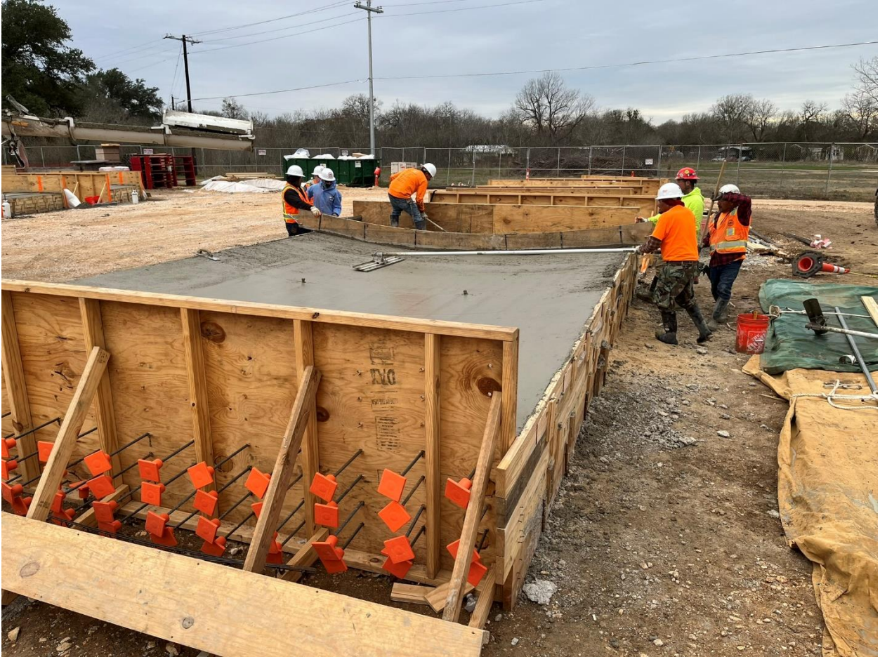
2J – Floating and finishing of concrete for Wall Panel pieces.
