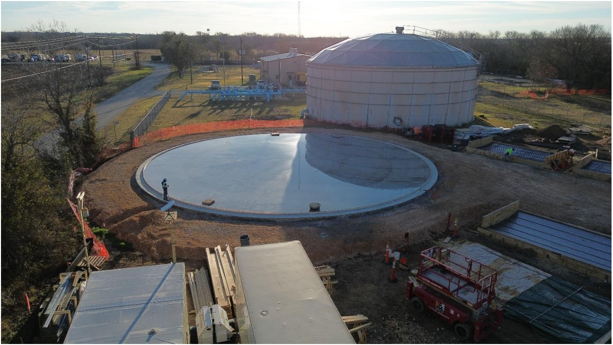
2E – Aerial side view of completed concrete pour at Tank Floor Structure (submerged in water for cure).
