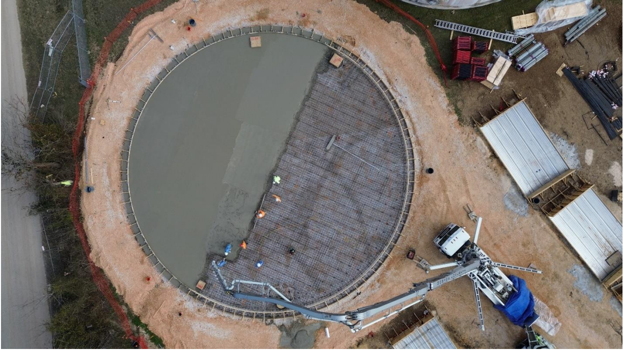
2A – Concrete Pump Truck delivering concrete to Tank Floor Structure.
